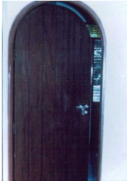
Figure 1.4i7 composite door (Source : comptec, I.I.T. Madras)
